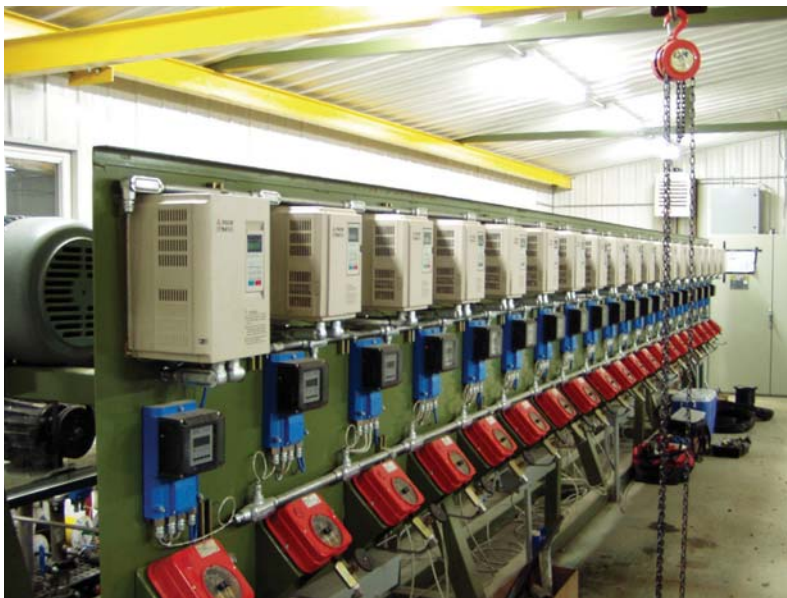
Figure 2. Each pump serves a separate oil well. Pump flow and pressure are regulated via VFD speed control in response to conditions in the well.
