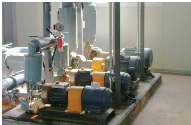
Figure 5. Installing seal-less Hydra-Cell pumps removed leak problem and halved energy use at Seonam.
