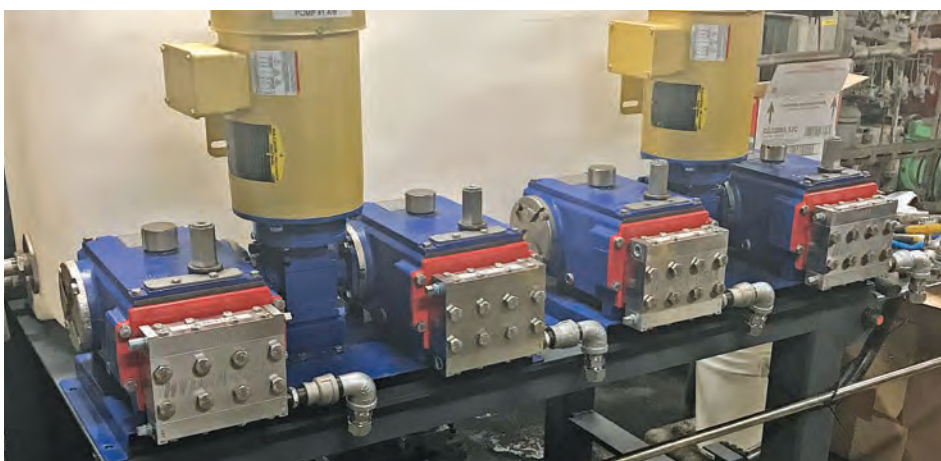
Chemical boiler feed at a power plant. Four MT8 pumps running off two gearboxes and two motors shows its duplexing capability.
