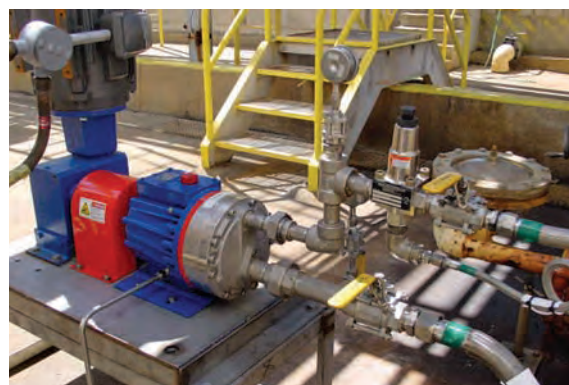
P600 used to inject Ammonia. Shown with a Hydra-Cell C62 pressure regulating valve.
