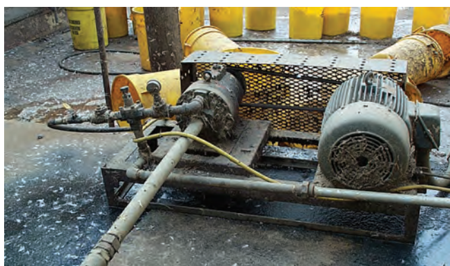
Hydra-Cell used for high-pressure cleaning in a poultry processing plant.
