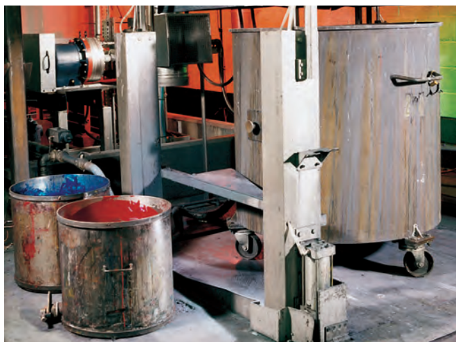
Hydra-Cell installation for cleaning paint containers.
