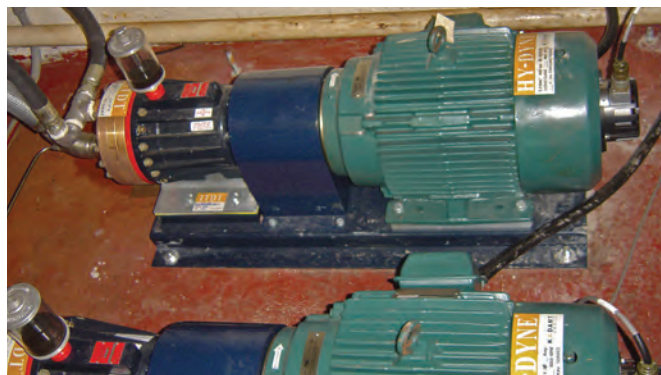
High-pressure shower application for Hydra-Cell at a paper mill.
