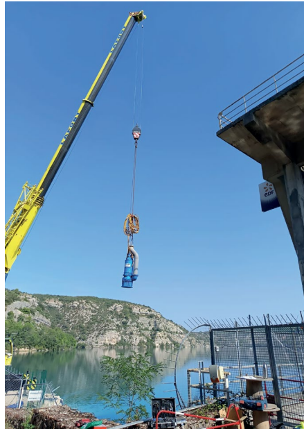
A pump being lowered into place. Picture from Tsurumi
