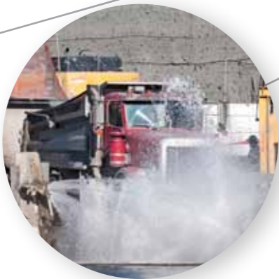
Construction site vehicle wash
